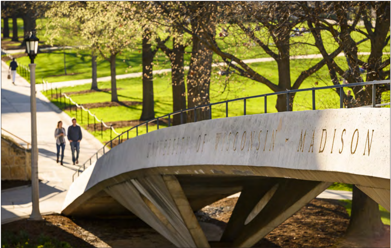
Park Street pedestrian bridge
